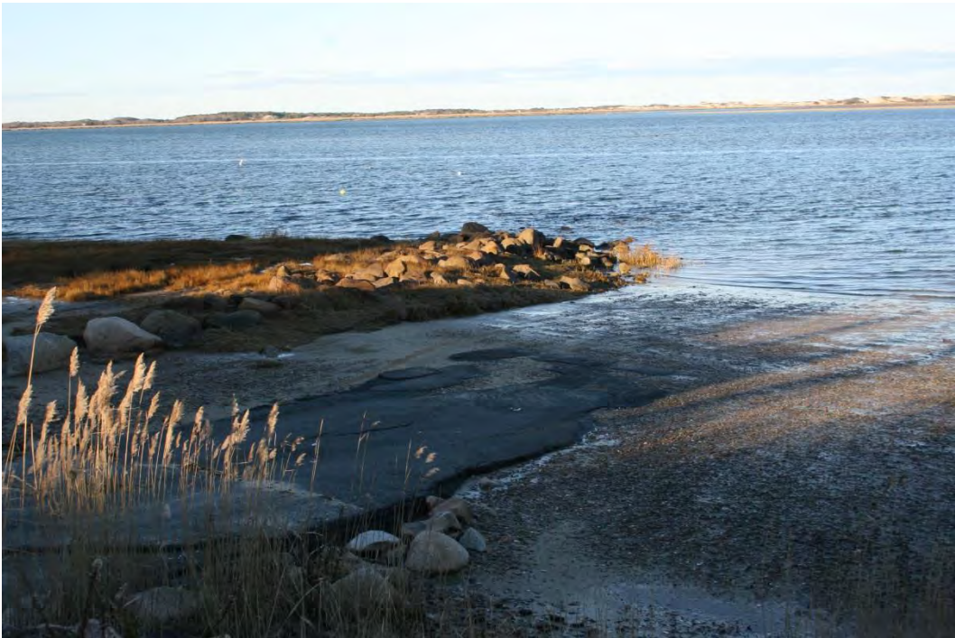
Scudder's Lane Boat Ramp
