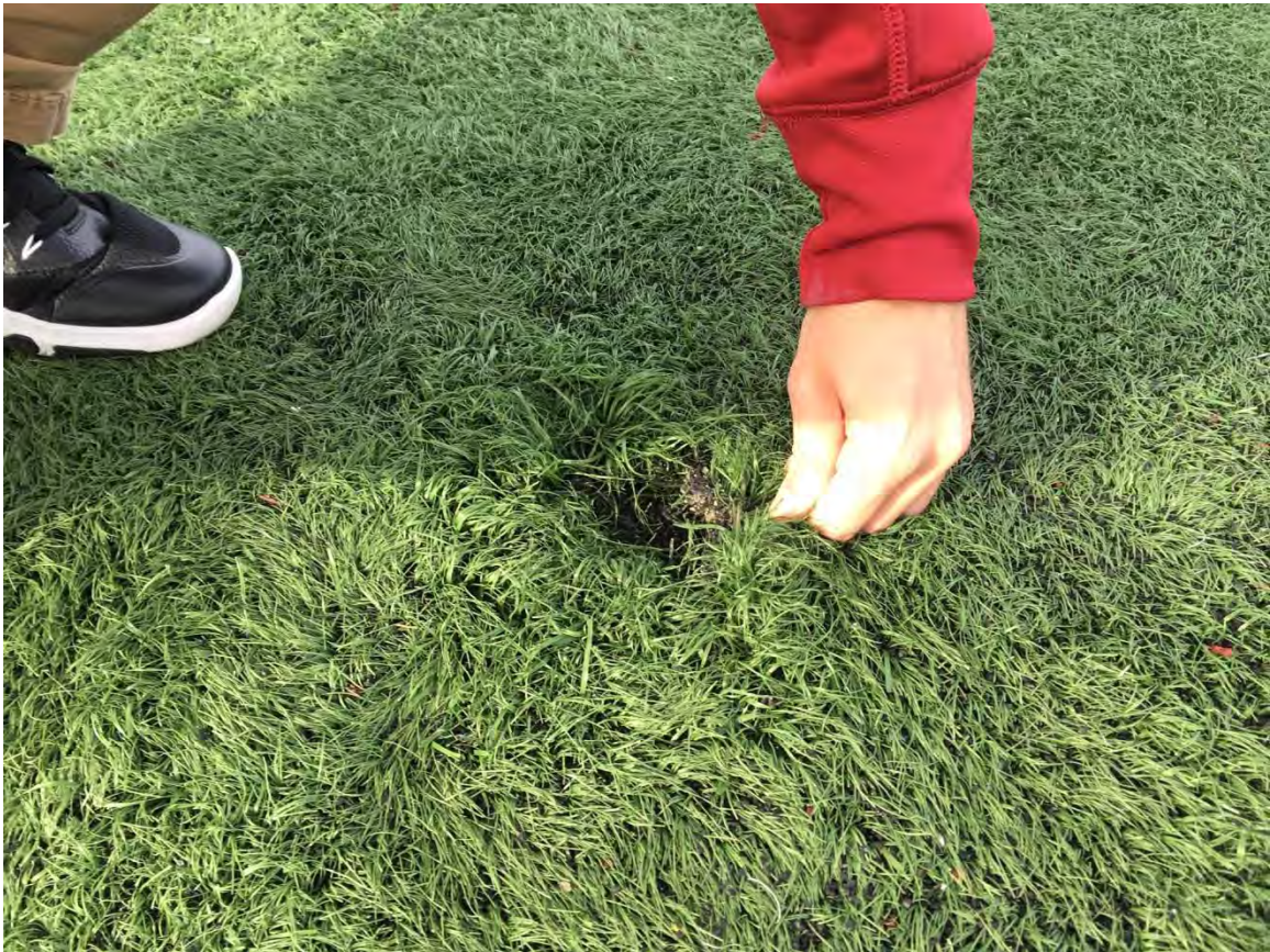
Barnstable High School Synthetic Turf Replacement
