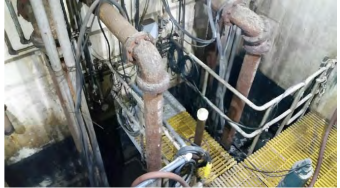
Old Colony Pump Station Wet Well
