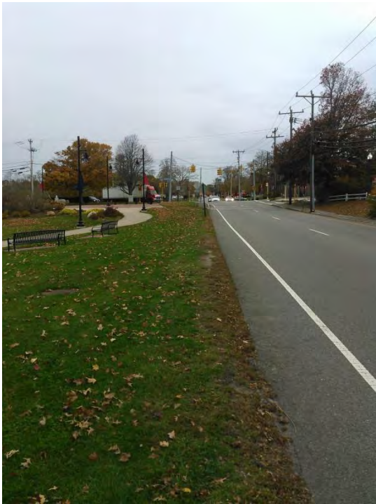
Sidewalk Installation: Bumps River Rd Centerville, Main St Cotuit, South St Hyannis
