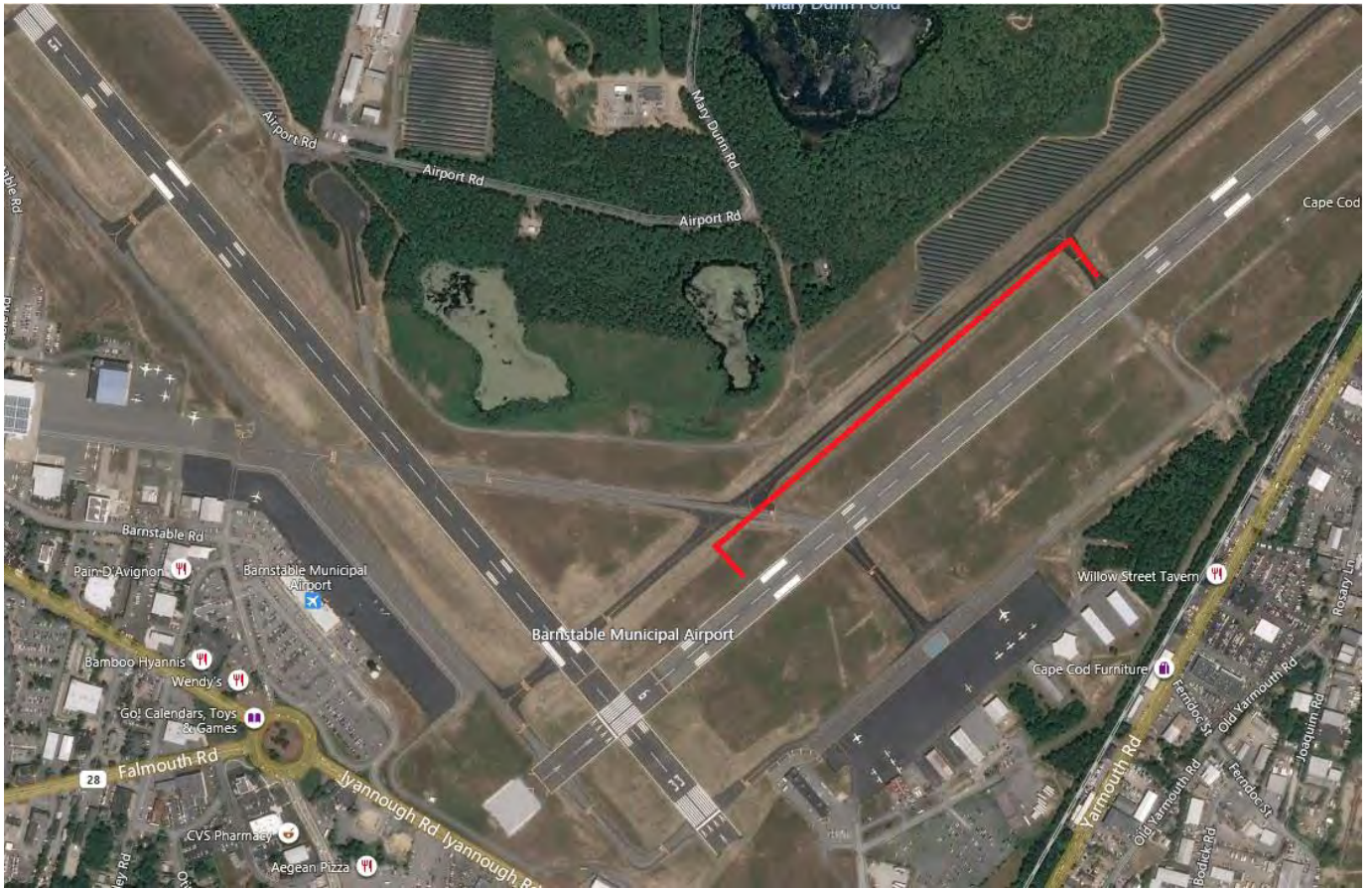
Portion of Taxiway Bravo
