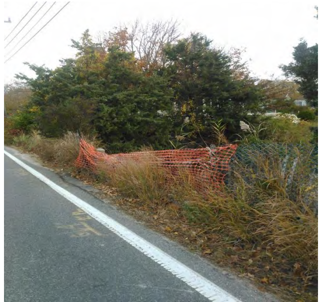
Snows Creek Culvert
