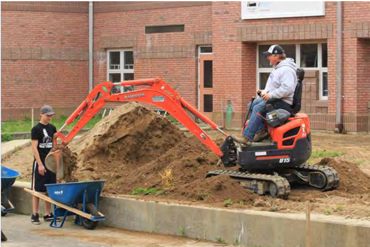
Barnstable Unit Elementary Courtyard Improvements
